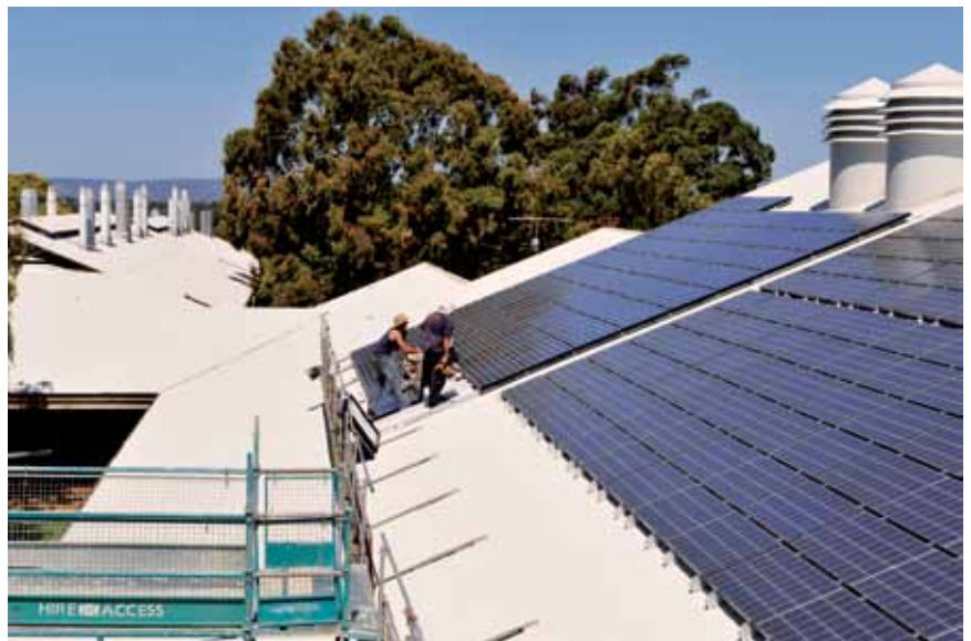
Installing solar panels on the library roof
